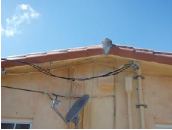
The service wires should be improved.
