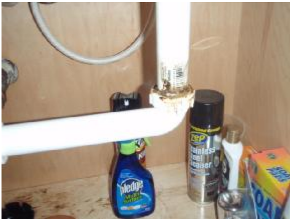
Tighten the sink trap
