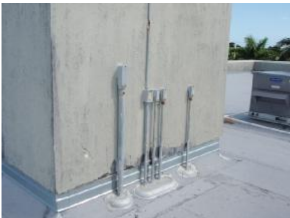
View of the proper flashing.
