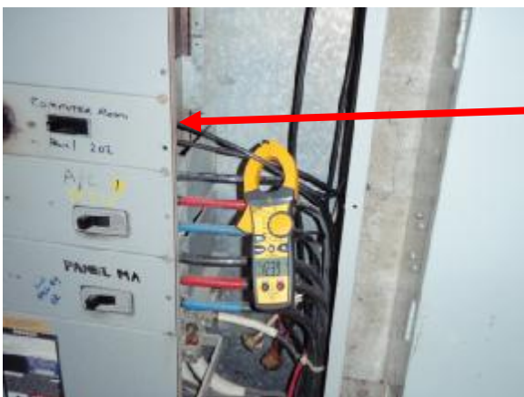
This leg is unbalanced and extremely overheated.
