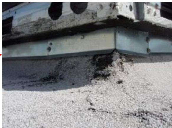
The well flashed curbs.
