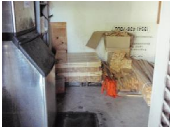
View of the exterior storage room.
