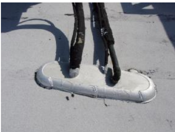
Well flashed roof penetrations
