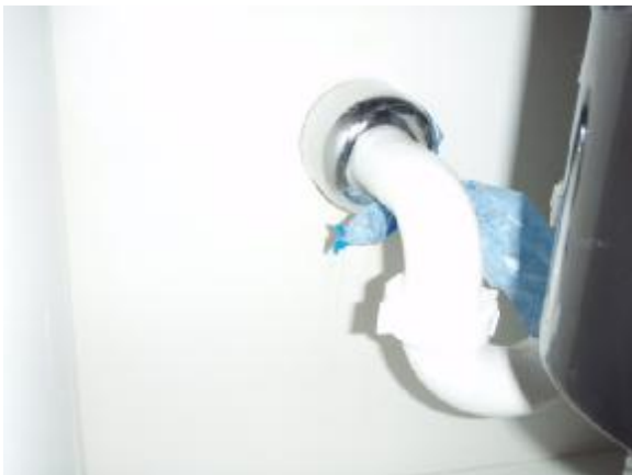
The trap below the kitchen is taped and drips water.
